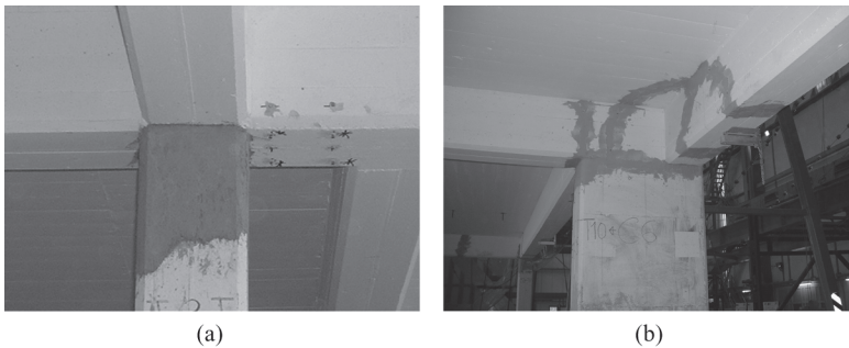
Figure 7 – Columns C3 (a) and C6 (b) at 1 st story after restoration of original cross-sections
